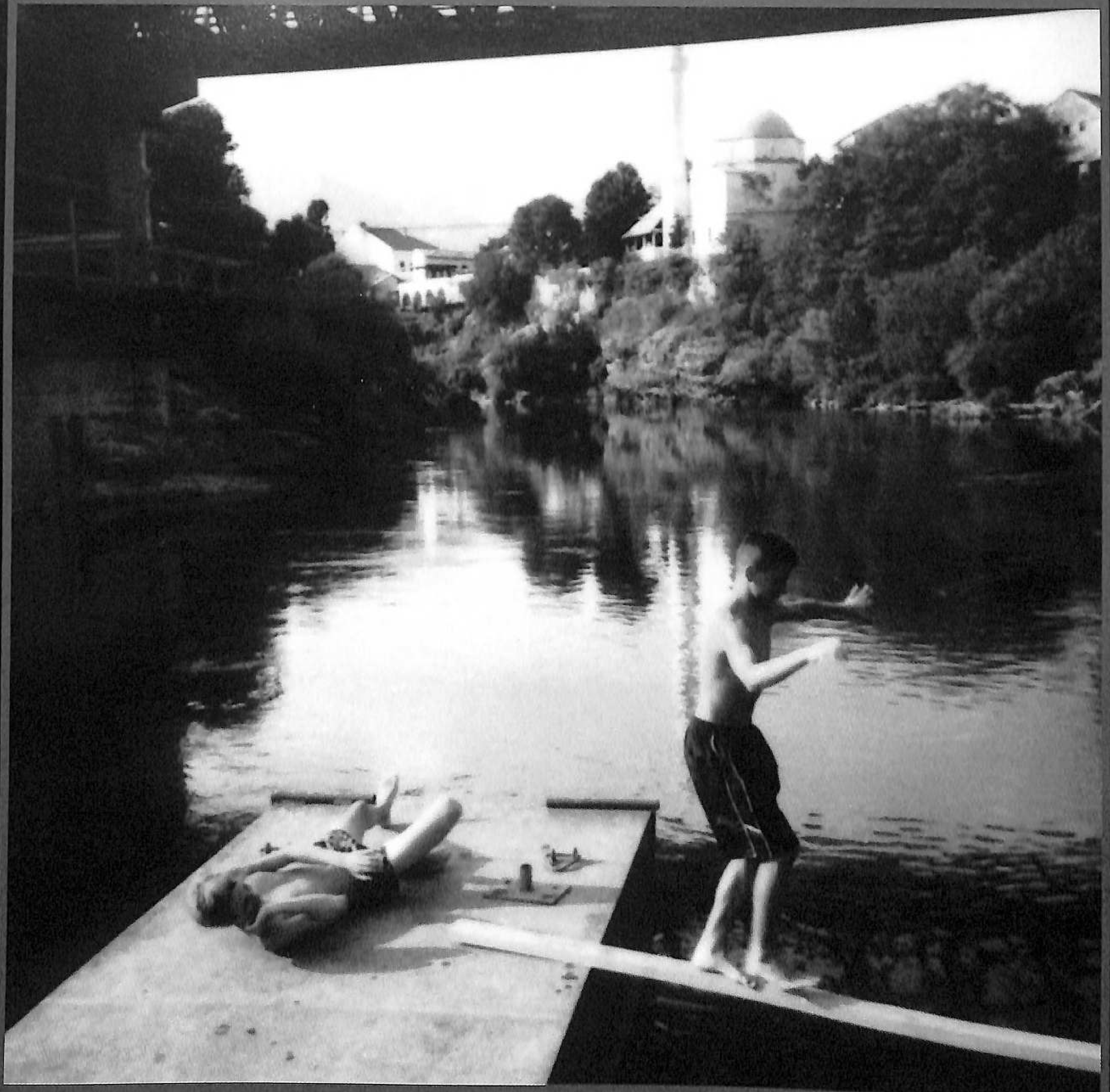
On the bridge at Mostar, which was being rebuilt. August 2003.
